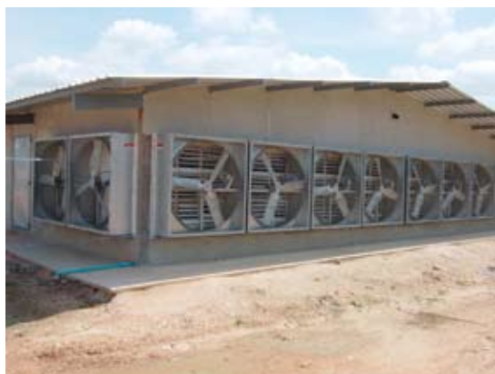
Figure 4.3: Example of power ventilation
