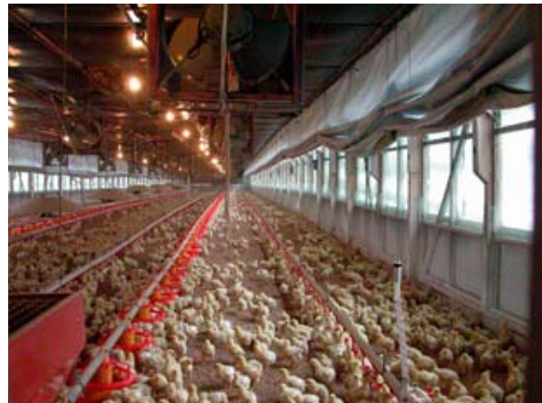
Figure 4.2: Example of natural ventilation
