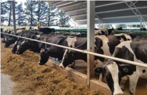
Post and rail barriers Relatively inexpensive. Can be adjustable.
